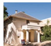
44. Old Court House Law Museum, Stirling Gardens, cnr Barrack Street & St Georges Terrace
